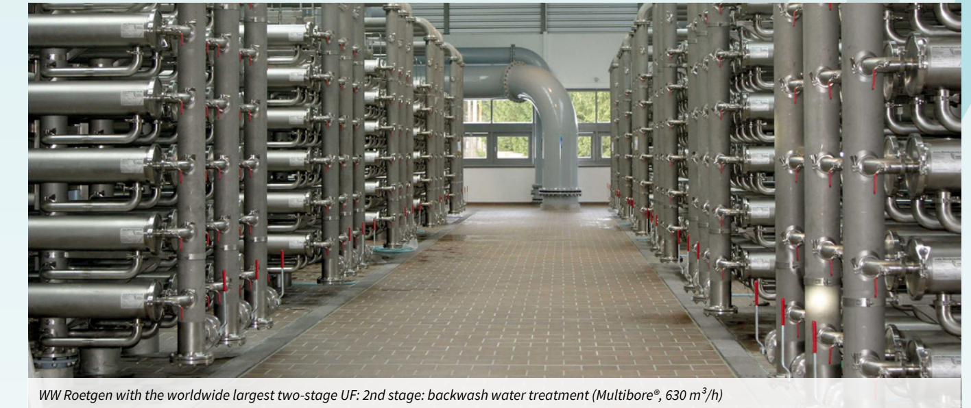
WW Roetgen with the worldwide largest two-stage UF: 2nd stage: backwash water treatment (Multibore®, 630 m 3 /h)
